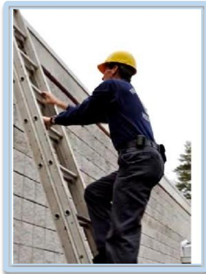
In the photo above, the worker is safe because the base of that 20 foot ladder is 4 feet (or  $\frac{1}{4}$  of the working height) away from the 16 foot wall.
